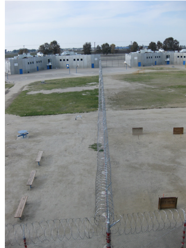
Figure 4 – New Security Fence
