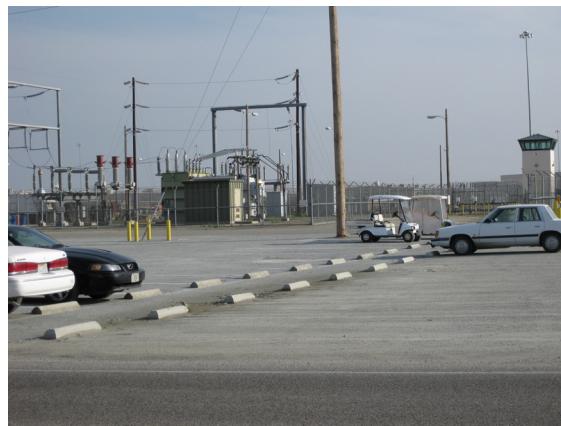
Figure 1 – Recently renovated parking lot
